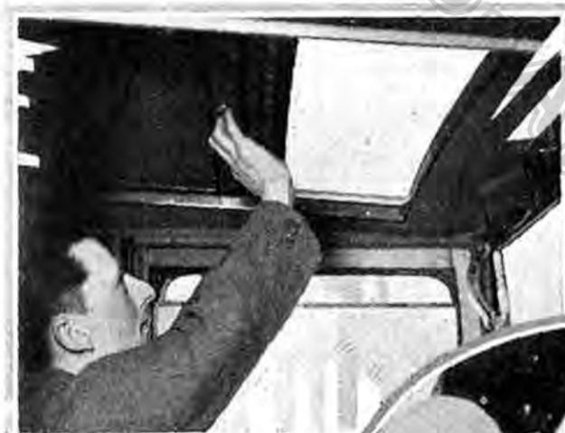
Above is the easily-operated Fytchley sliding roof, and on the right we see one of the cubby holes, which now have covers. A larger one still is available on the passenger side of the car.
