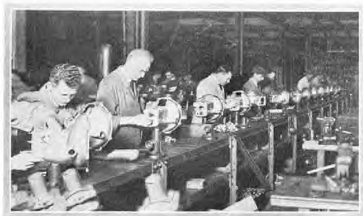
A general view of the gearbox assembly line. Here again a conveyor track and special fixtures to expedite the work are employed.
