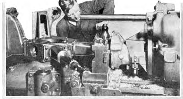
The gearbox housing is undergoing the necessary machining operation on this specially equipped high capacity cupstan lathe.
