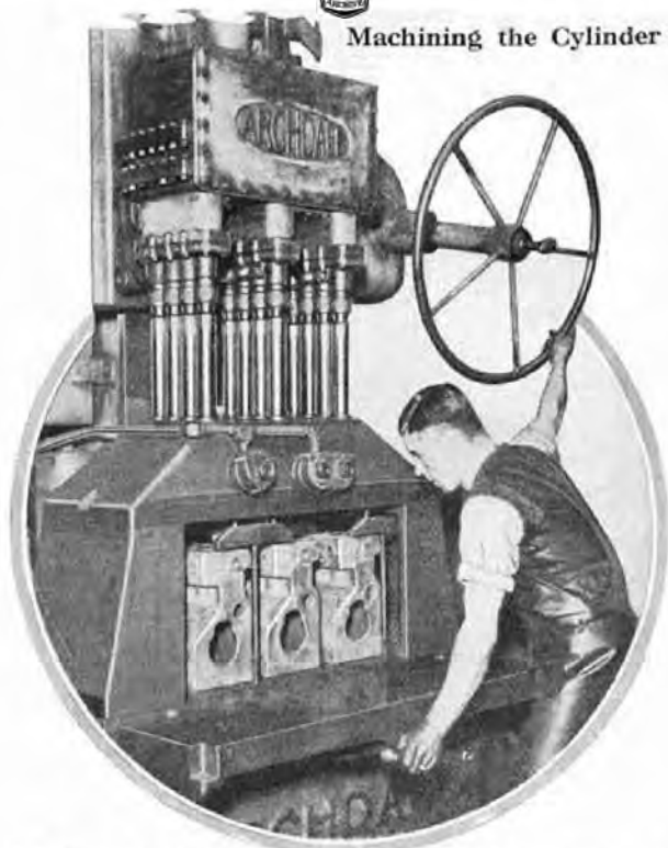
Boring Minor cylinder blocks on the special multiple boring machine.
