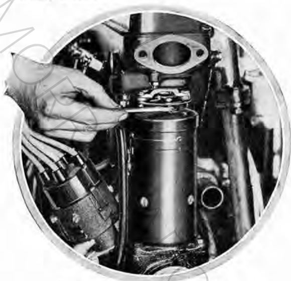
Removing the coupling bolts of the flexible coupling.
